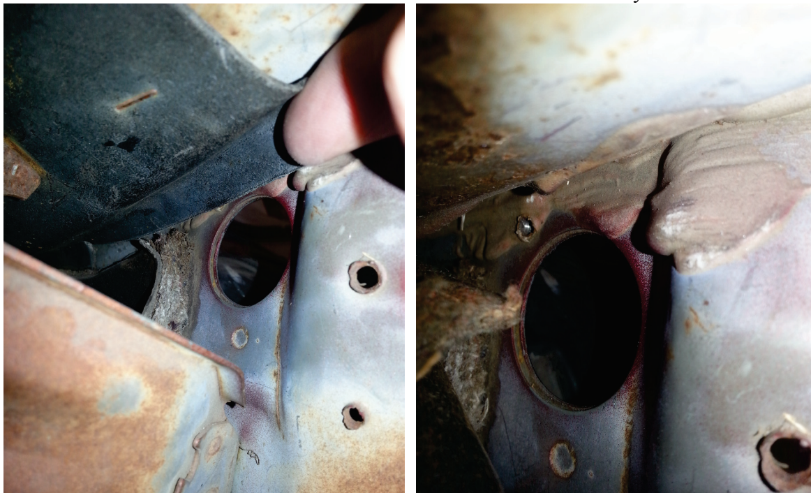
Shown are the insulation liner and excess sealant. Remove.
