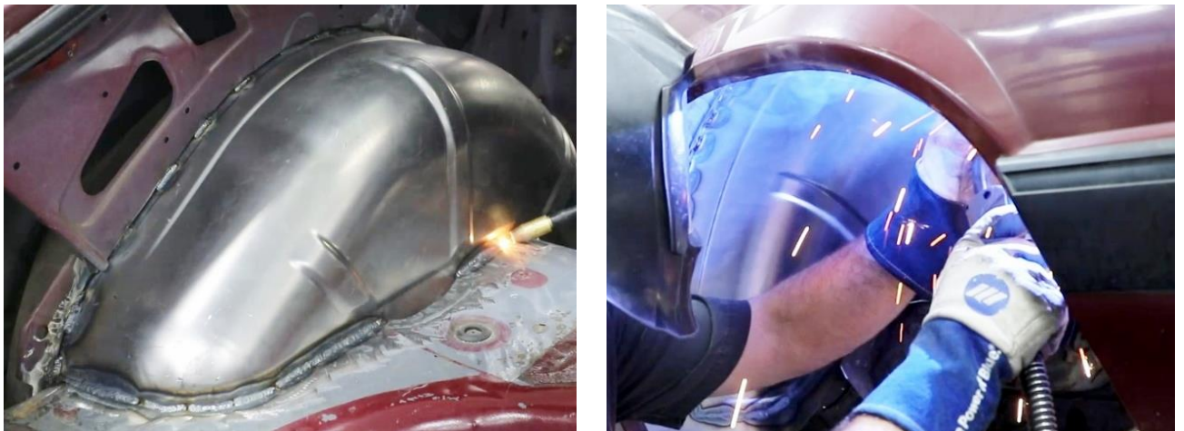
Figure 40 - Finish Weld around Mini-Tub
