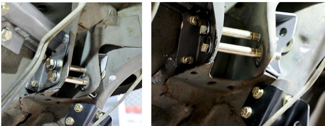
Figure 52 - Verify Installed Hardware
