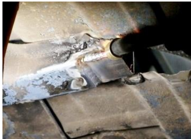
Figure 43 – Weld Back of Connector
