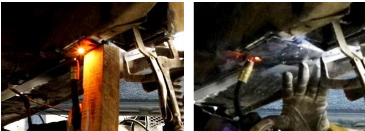
Figure 50 – Weld Doubler Plate
