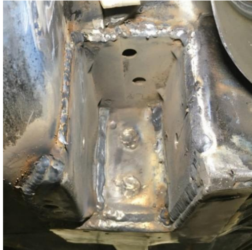
Figure 54 – Weld Factory Sheet Metal
